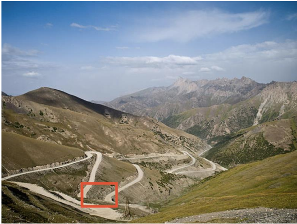
Fig. 2.3. a) Taldyk pass in 2008 before construction. (Source: Wikipedia)
