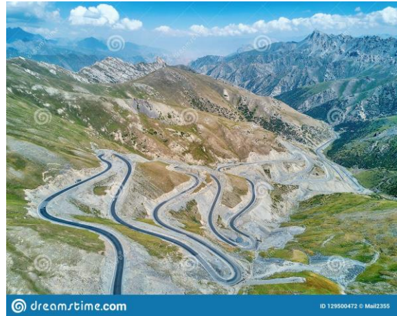
Fig. 2.3. b) Taldyk pass in 2018 after construction with heavy excavations in the slope. (Source: dreamstime)
