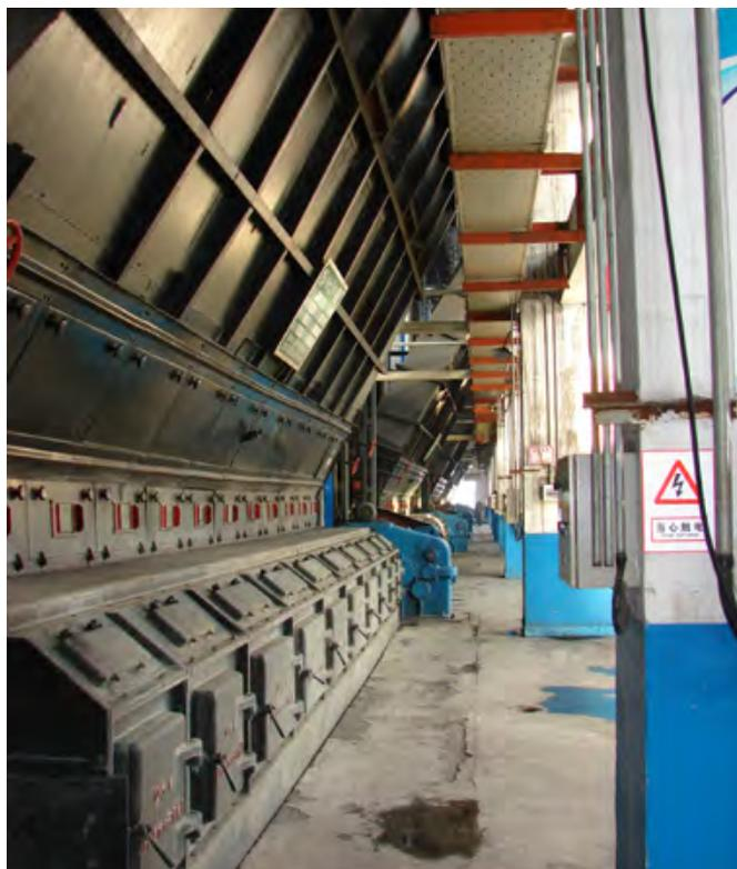
8 units of 70 MW high temperature hot water boilers and auxiliary engines installed in the project.
